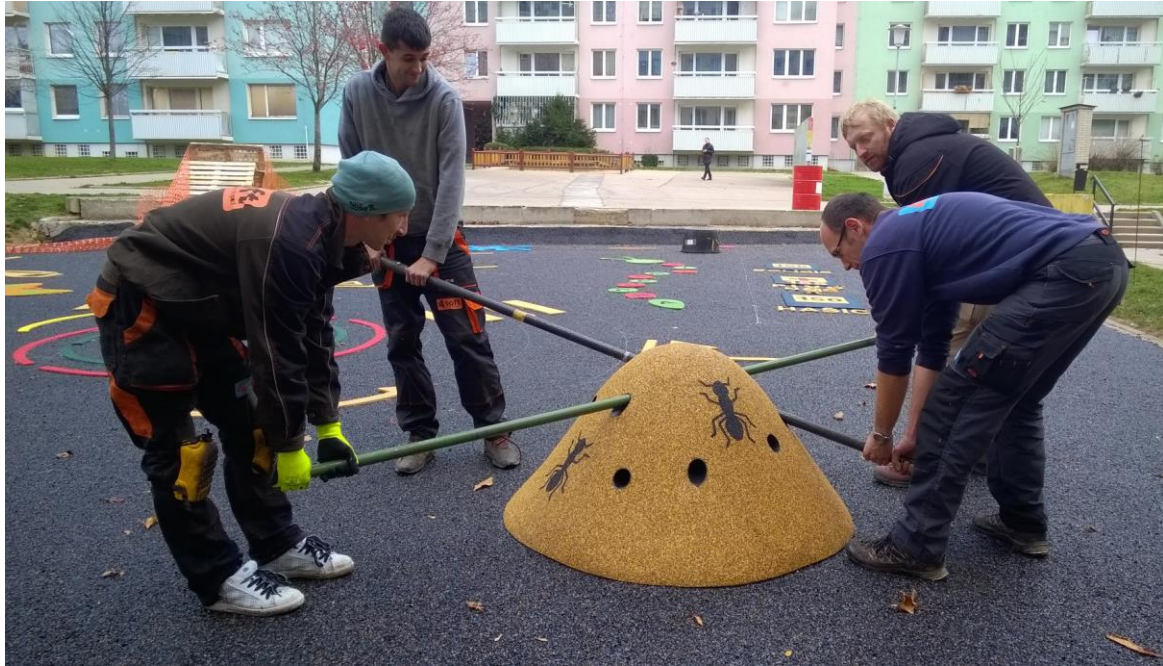
To transport heavy 3D anthill use two iron sticks to pass them through the holes.
